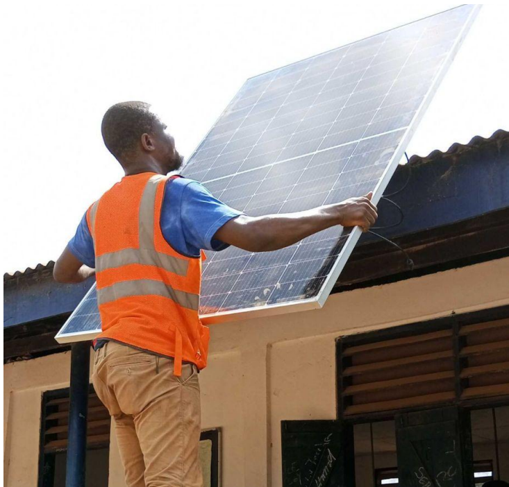
A solar panel installation. Photo courtesy of Rising Academy Network.
